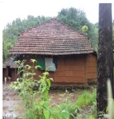
Tribal home made by dry stems of Strobilanthus spp.
